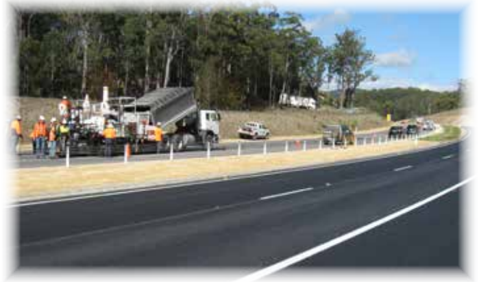
SAMIfalt A15E (in an SMA 10 mix) Pacific Highway, Coopernook, NSW
